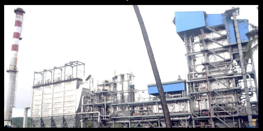
18 TPH, 45 Kg/cm<sup>2</sup>g, 400°C Slop with Imported Coal as supporting fuel
